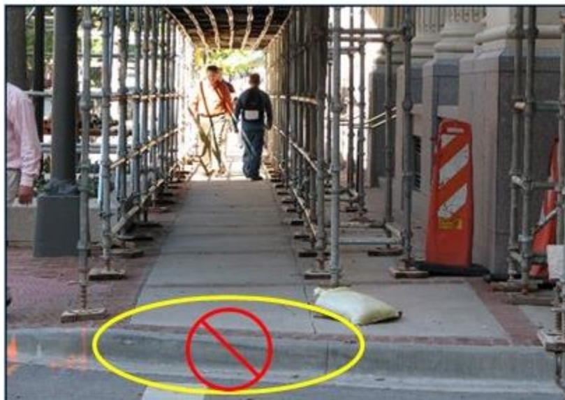
Proper Temporary curb ramps are required wherever the diversion path traverses a curb (Source: J. Barlow, Accessible Design for the Blind)
