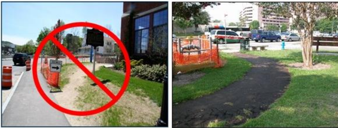
Diversion paths should be smooth, solid, weather resistant, and detectable by visually impaired pedestrians. (Source: J. Barlow, Accessible Design for the Blind)
